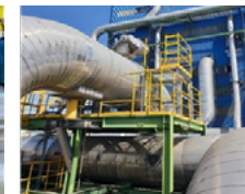
Installation of K-301 and 302 inspection platforms
