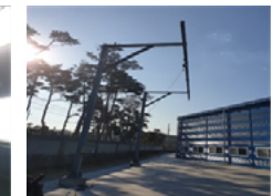
Installation of safety cradle for vehicle work
