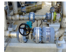
Installation of shatterproof cover for all HCl lines
