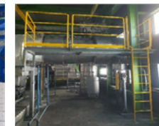
Installation of safety footrest for XV-4181 inspection
